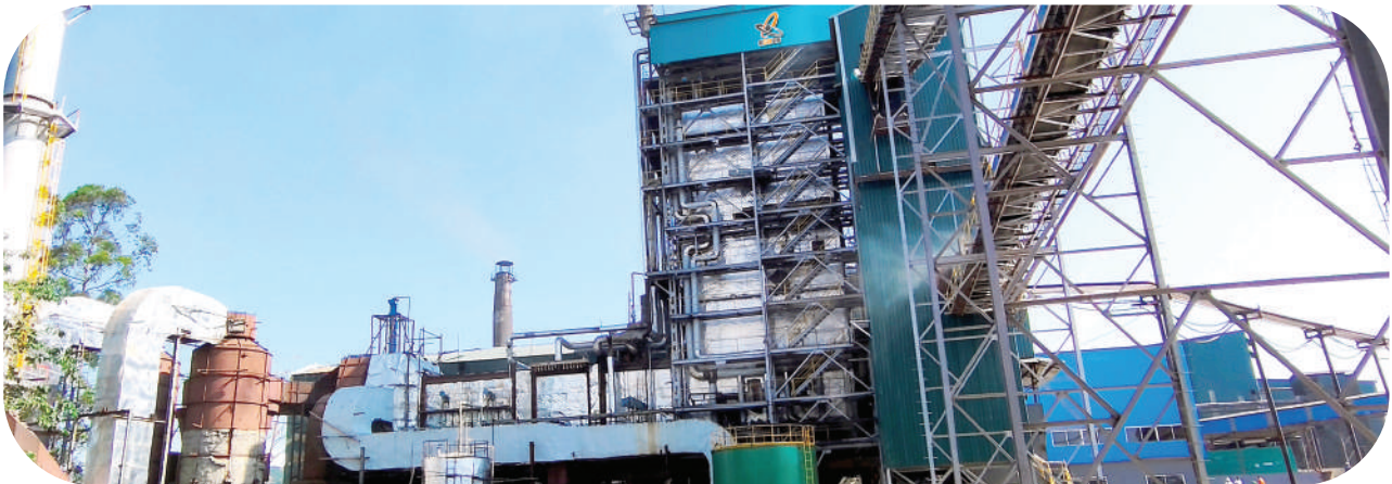
CPP Power Plant
